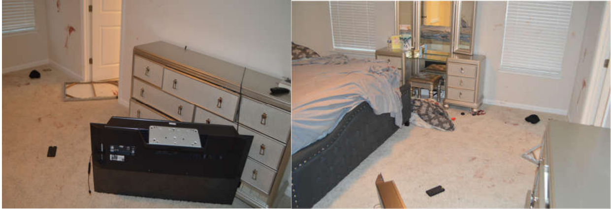
Figures 7 and 8. Photographs of the damage to the bedroom caused by the attack on [REDACTED]
